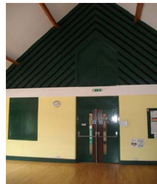
Figure: Loft void at end
