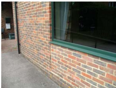
Figure: Double glazed windows with constructed wall replacement
