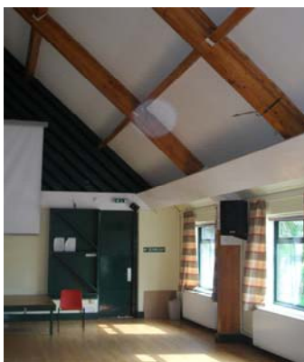
Figure: main apex ceiling and loft void
