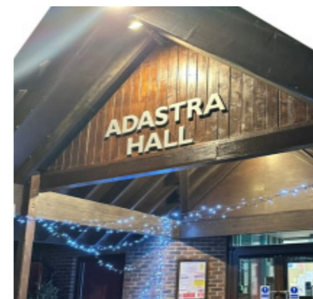
Refurbishment and signage.
